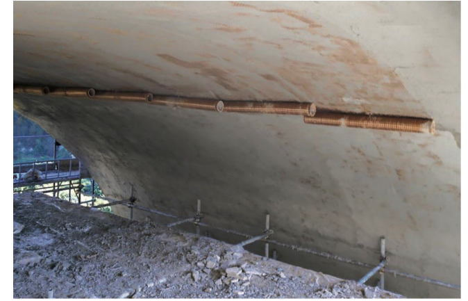
Masonry arch strengthening
