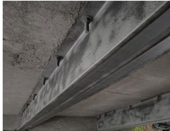
KY 32 Bridge, Kentucky: UHM CFRP Plates
