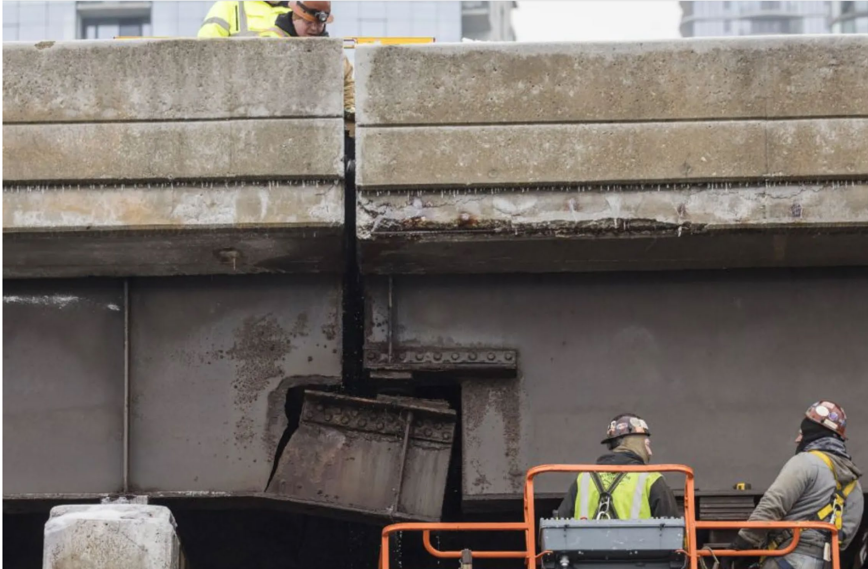
Northbound Lake Shore Drive bridge – Chicago (US) - 2022
