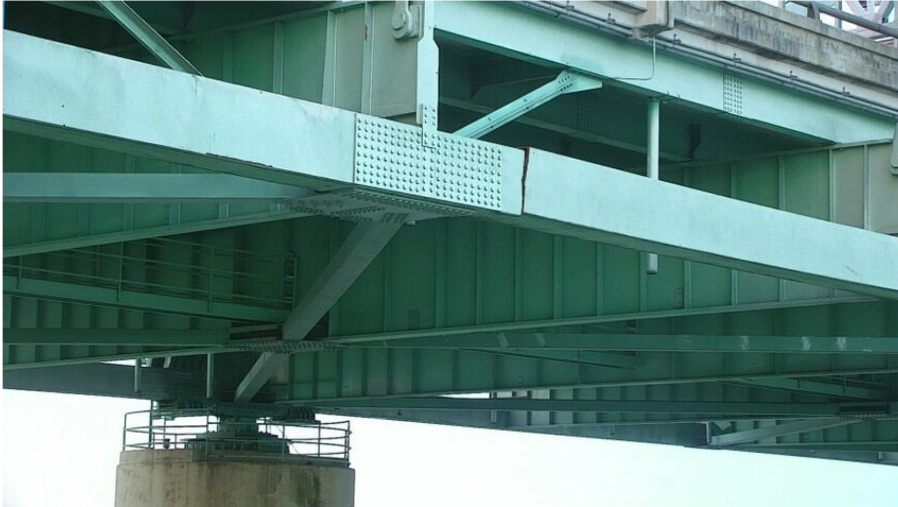
I-40 bridge – Memphis (US) - 2021
