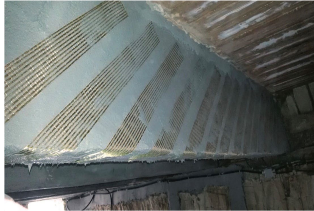
Shear strengthening of RC beams
