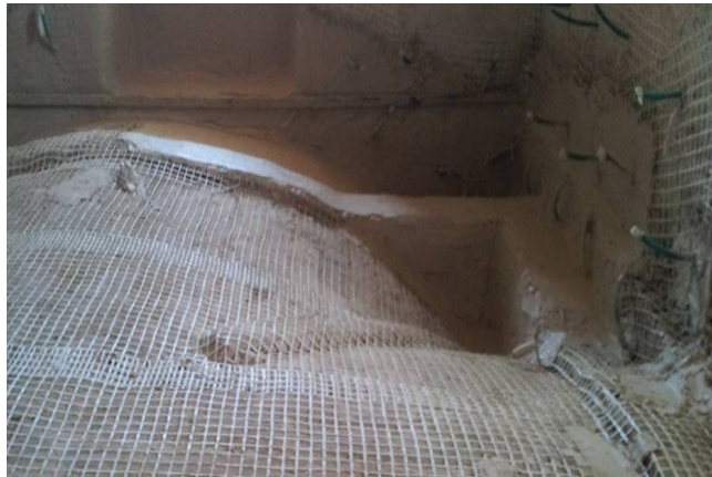
Masonry vaults strengthening
