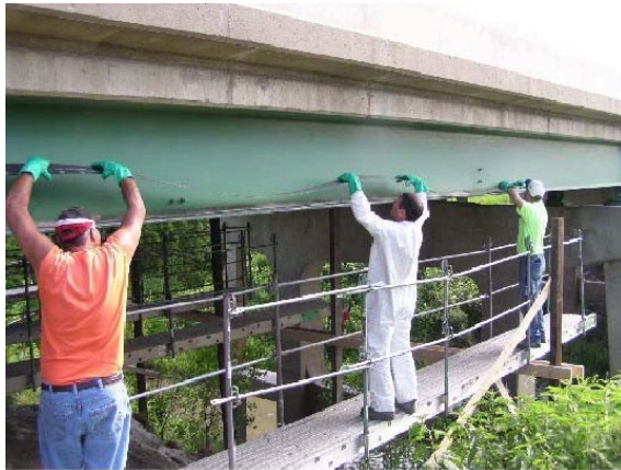
State Highway 92 bridge, Iowa (US): CFRP Plates
