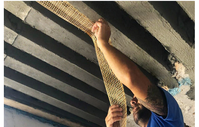
Flexural strengthening of slabs
